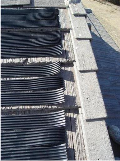
Assemble the manifolds at the other end to the fin tubes first, then to each other and secure to the roof using the same methods described. It's very important you don't try to glue the headers to each other first. . A chalk line can be helpful. Pay close attention that the fin tube doesn't shift. The glue (PL and PG) take a while to dry.
