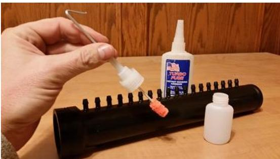
Tile roof installations can not be prefabbed. Take care gluing the fin tubes to the manifolds with the CA adhesive. It is important to fully wet the entire surface of the nipples before slipping the fin tubes on 2 tubes at a time. Strip the 6 tube wide fin tubes near the end so that you can work with 2 tubes at a time.
