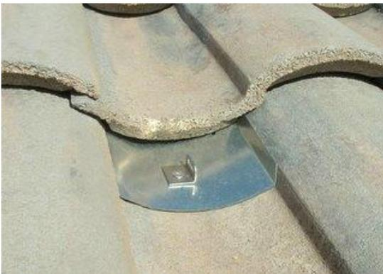
If necessary another method is to slip vinyl coated ss strap through a strap bracket as shown above left. Then just slip it between tiles (lift tiles with a screwdriver) so it catches in the space above the tile.
