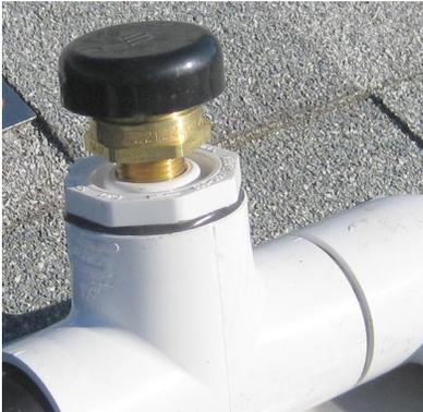
The vacuum breaker should be teed off the pipe entering the bottom corner of the bank of collectors. Use Teflon tape on the 1/2" threaded connection. Wrap the Teflon tape around the threads 5 times clockwise. The vacuum breaker sits vertically.
