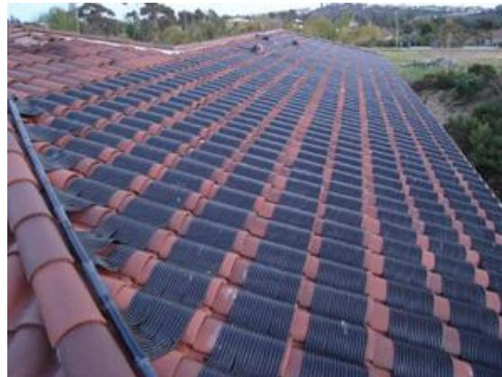
If the manifolds are angled it means there is more space between manifolds. You`ll need a glue-on PVC coupling for each male end to PVC pipe or you can alternate the directions where male ends are connected via pvc couplings and female ends are glued together via varying lengths of pvc pipe to line manifolds up so they correspond to the fin tubes row by tile row. For more on corners and angled headers refer to the general installation manual. SEE drawing TILE1000
