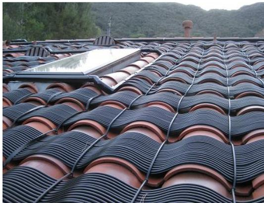
Use regular solid black vinyl coated electrical wire (12 gage). Cut pieces about 8" long, bend one end 90 degrees, lift tile with a screwdriver, slide the bent end between tiles until you can rotate the wire 90 degrees so it grabs the top of the tile below. This wire can secure the one or two tube wide strip. Use needle nose pliers to bend the wire. This positions and secures all the fin tubing. You can glue it all down later for best
